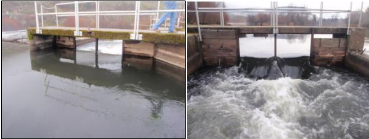
Figure 4-3. A view downstream at the fish ladder flow control structure with 3,800 cfs total flow in the river (left). The right photo is an upstream view at the upper end of the fish ladder showing the variable control weir structure with adjustable boards.
