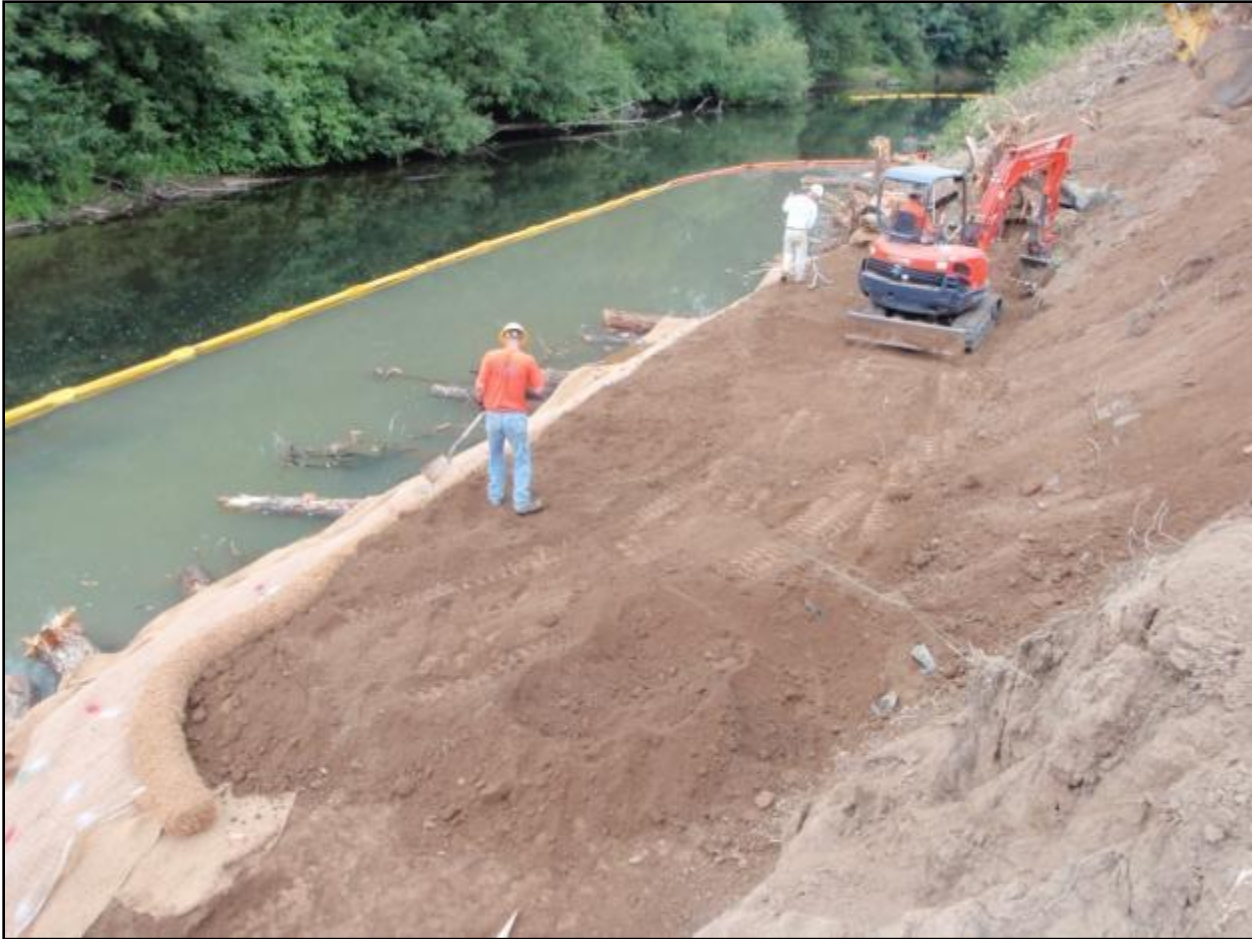
Figure 5-2. Example of a silt curtain isolating an active work area from clean water flowing by the project site. Turbid water contained within the work area by the silt curtain.
