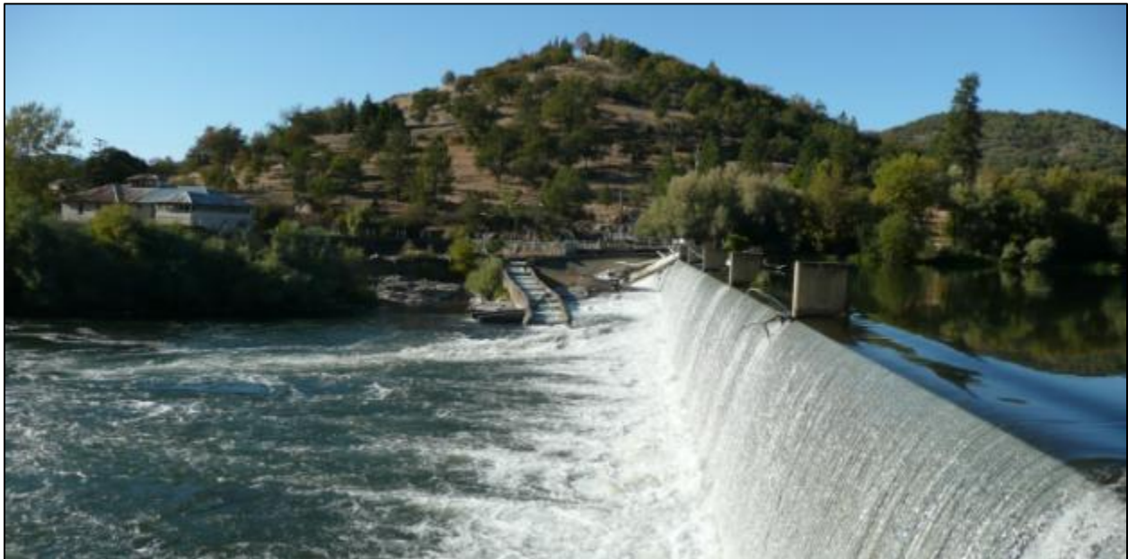
Figure 3-2. Existing view of Gold Ray Dam and fish ladder with total flow of 1,310 cfs.
