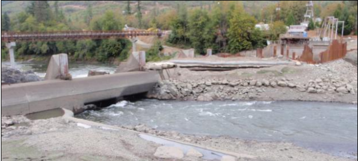
Figure 4-6. The Savage Rapids dam removal project showing 1,300 cfs going through radial gates with an average velocity of 6 fps and channel width of less than 60 ft.
