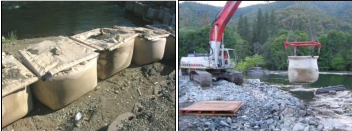
Figure 5-1. Example of bulk bags (left) and gravel cofferdam (right) used in combination for work area isolation on Savage Rapids dam and Gold Hill dam removal projects.
