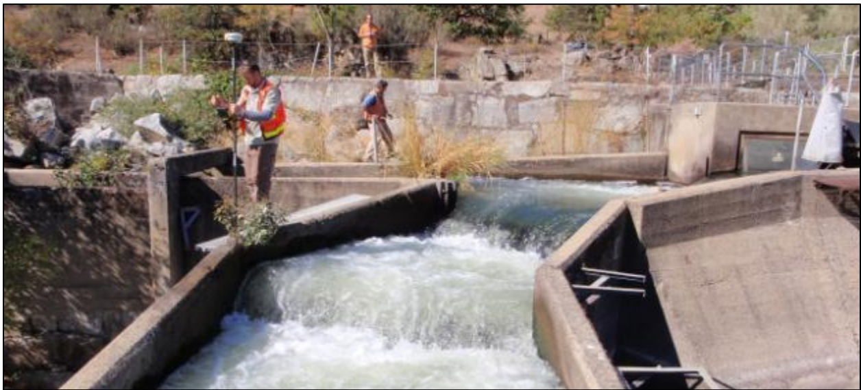
Figure 2-1. Surveying the existing fish ladder with a survey-grade GPS and total station.
