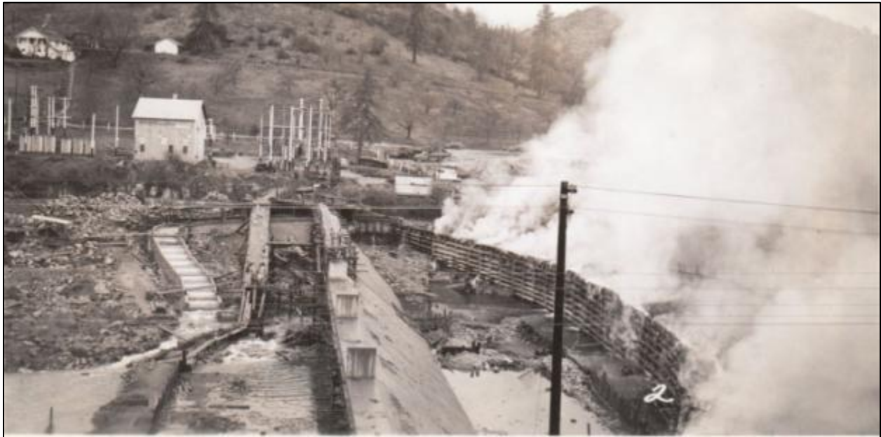
Figure 3-1. 1941 photo of concrete dam being built along with fish ladder and burning of the log crib dam. (photo courtesy of PacifCorps historical records)
