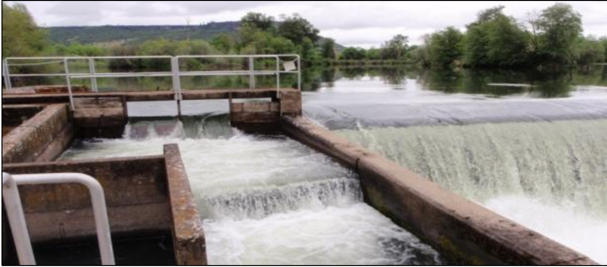
Figure 3-4. Looking upstream at the fish ladder flow control structure with 3,800 cfs total flow in river.
