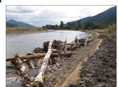
CONSTRUCTED ENGINEERED LARGE WOOD STRUCTURE
