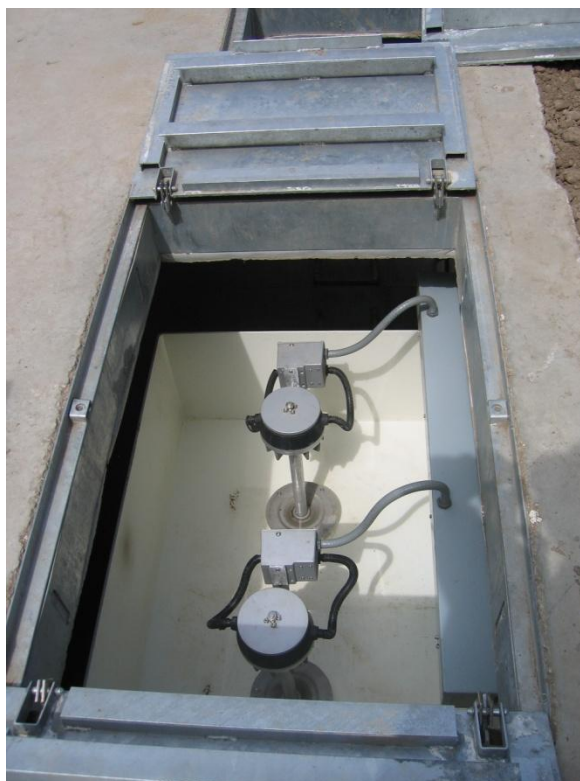
FIGURE 9: TWO LH1000 TURBINES INSTALLED IN A VAULT (ES&D, 2010)
