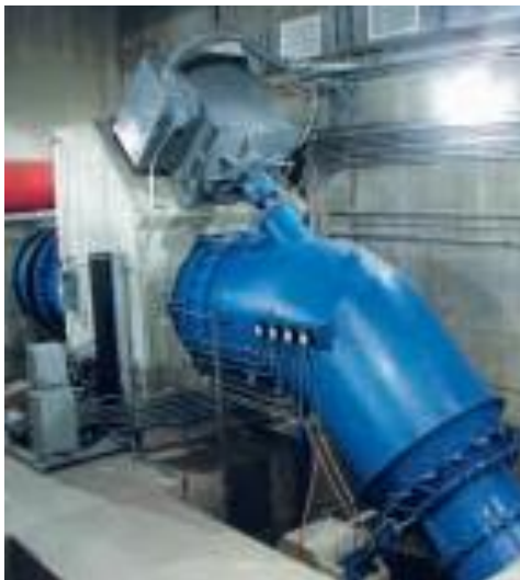
FIGURE 14: 300 KW KAPLAN TURBINE INSTALLED IN LOGAN, UTAH
