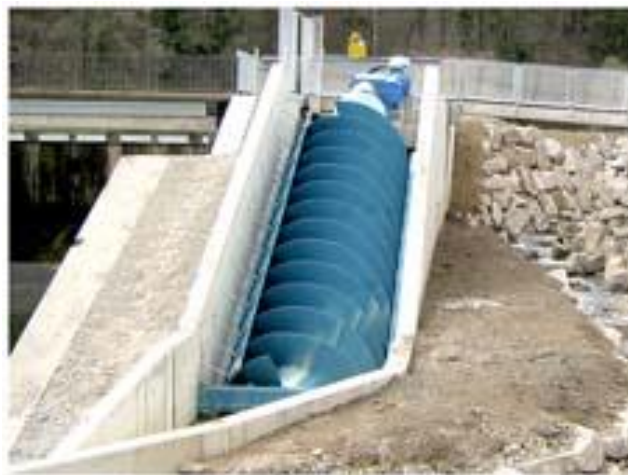
FIGURE 29: HYDRODYNAMIC SCREW (WWW.RITZ-ATRO.DE)
