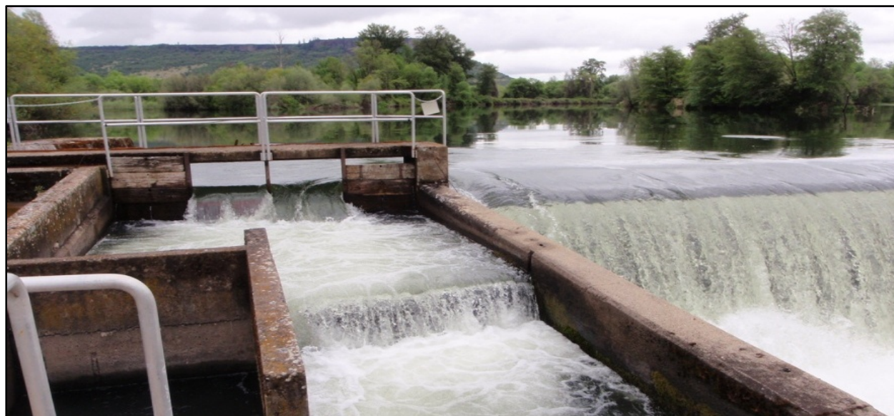
Figure 10: Looking Upstream at Fish Ladder Flow Control Structure with 3,800 cfs Total Flow in the River
