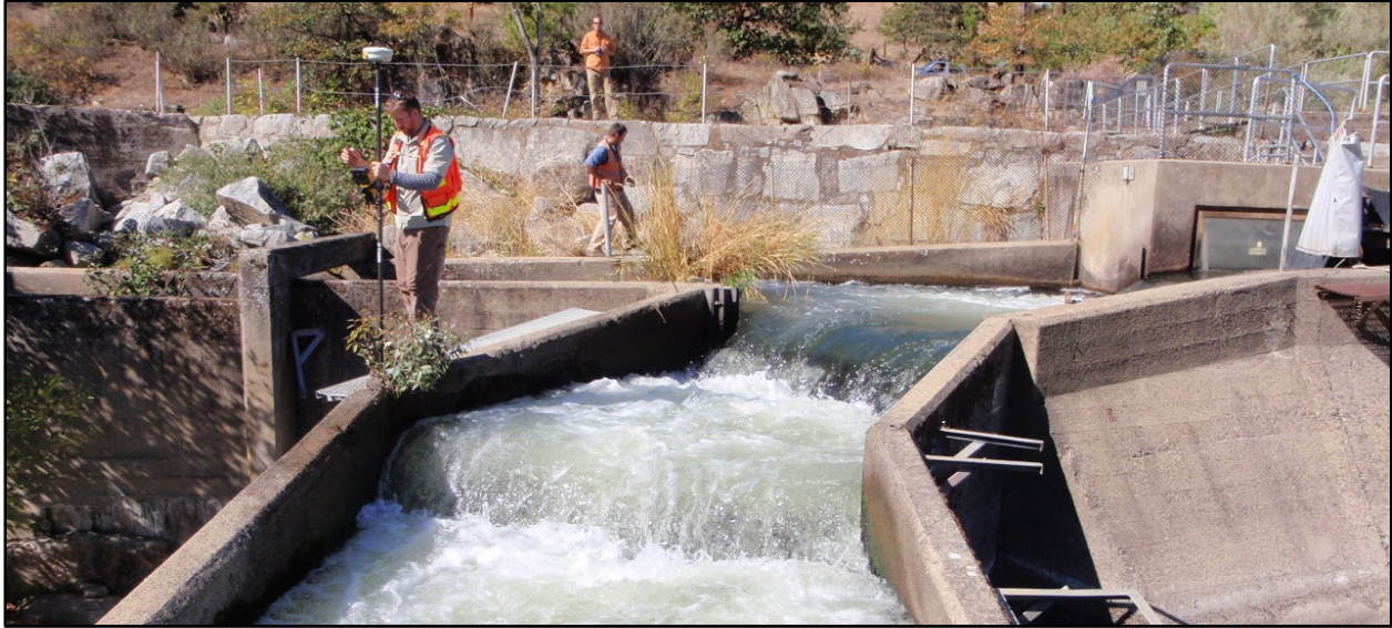
Figure 9: Surveying the Existing Fish Ladder with a Survey-grade GPS and Total Station
