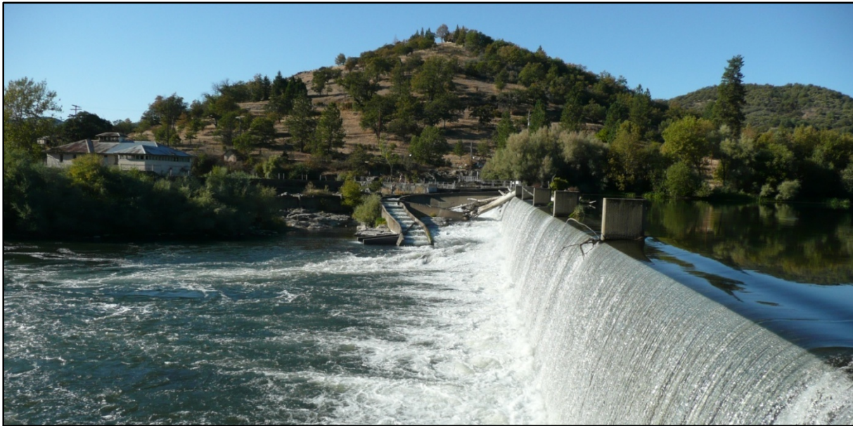
Figure 3: Existing View of Gold Ray Dam and Fish Ladder with Total Flow of 1,310 cfs
